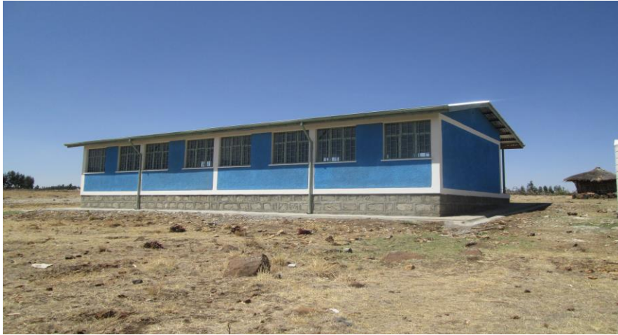
Fig 10: The new building at Workegur Elementary School.
