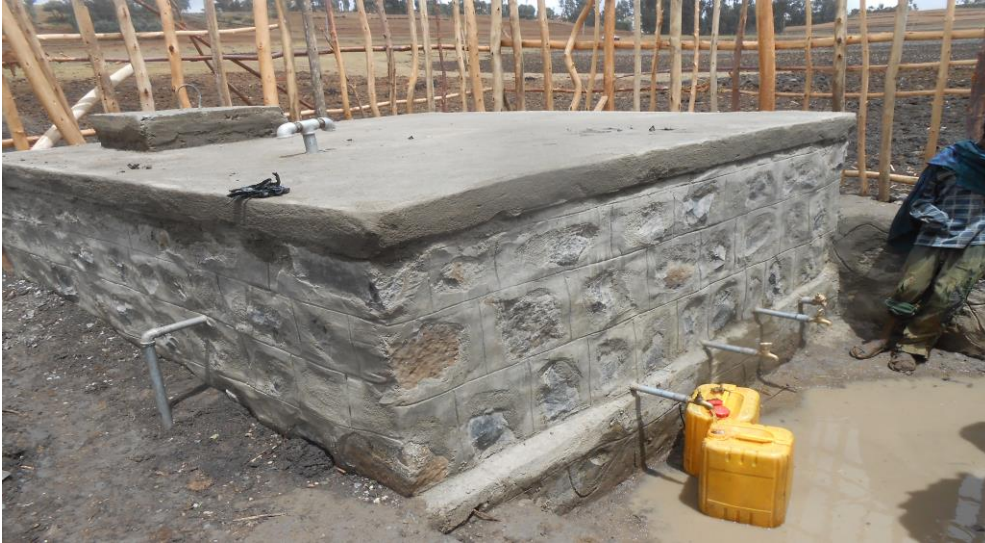
Fig 9: Water supply at Chenbirre
