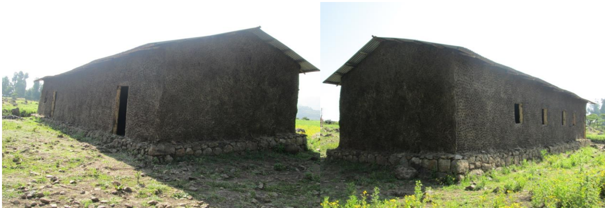
Fig 1: Rehabilitated FTC at Moyi
